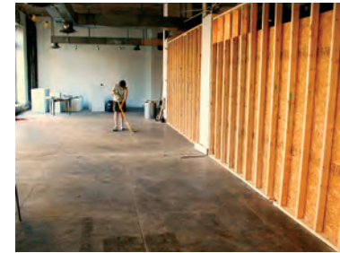
Constructing the new museum in the Book Building, downtown Detroit, 2001.
