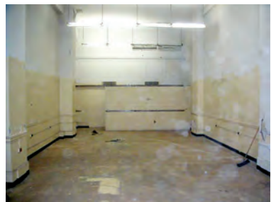
ArtCore: one of five Detroit galleries before renovation.
